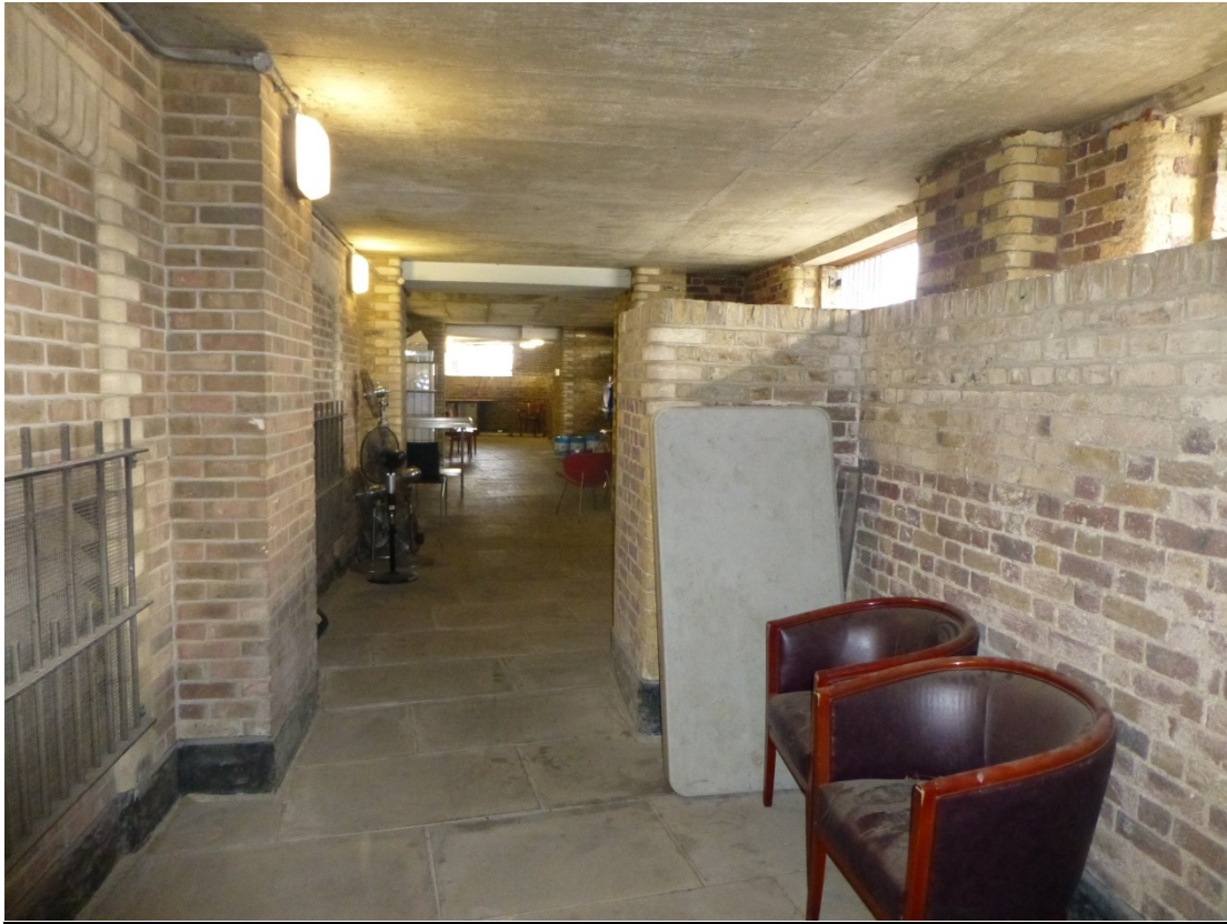
East-west section of covered walkway
